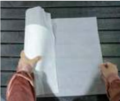
2. Wrap the substrate with a piece of protective paper;
